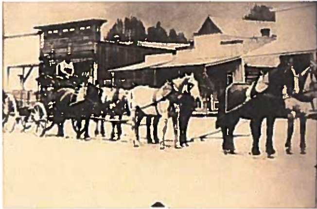
Hauling from the Minnie Moore Mine (Bellevue): Photo credit – The Community Library Center for Regional History
